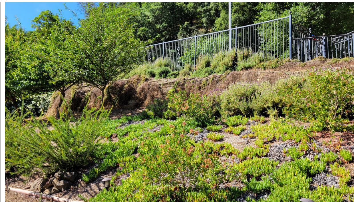
Photo 3. View of front of wall, facing south.
