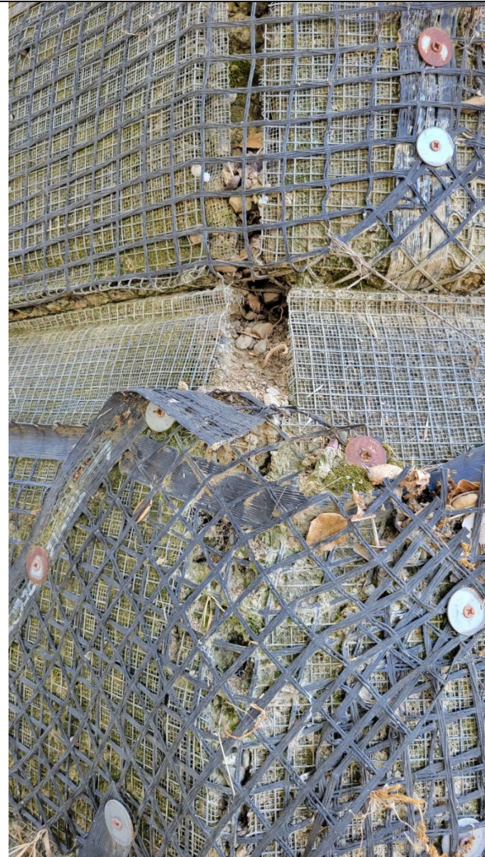
Photo 10. Geogrid anchorage at corner.
