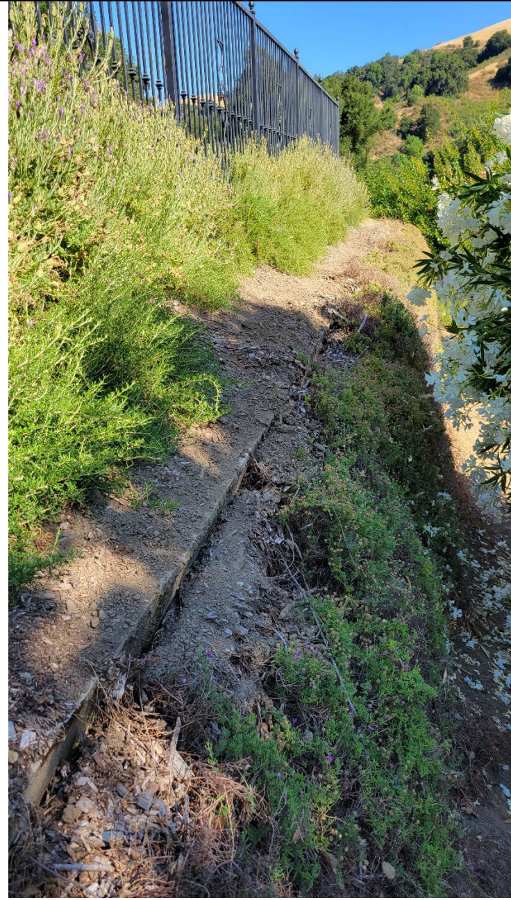
Photo 12. Close-up of top of wall, looking west.
