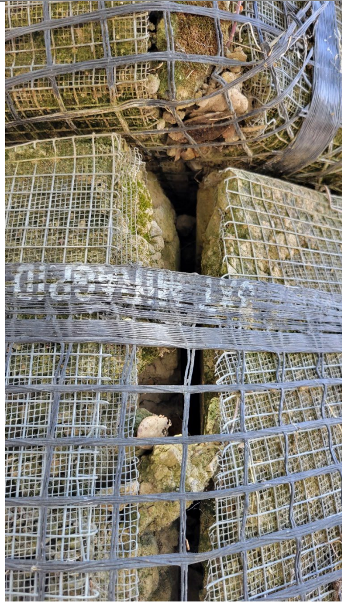
Photo 8. Cut corner units.
