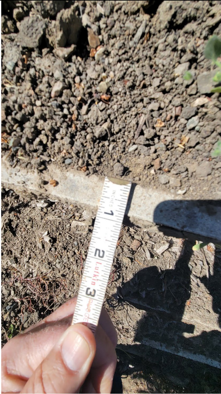
Photo 11. ¾-inch thick precast concrete face planter panel.
